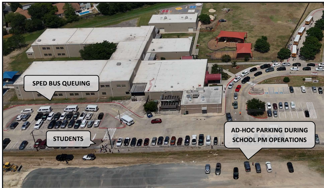
Figure 12 – Construction Area Ad-Hoc Parking
