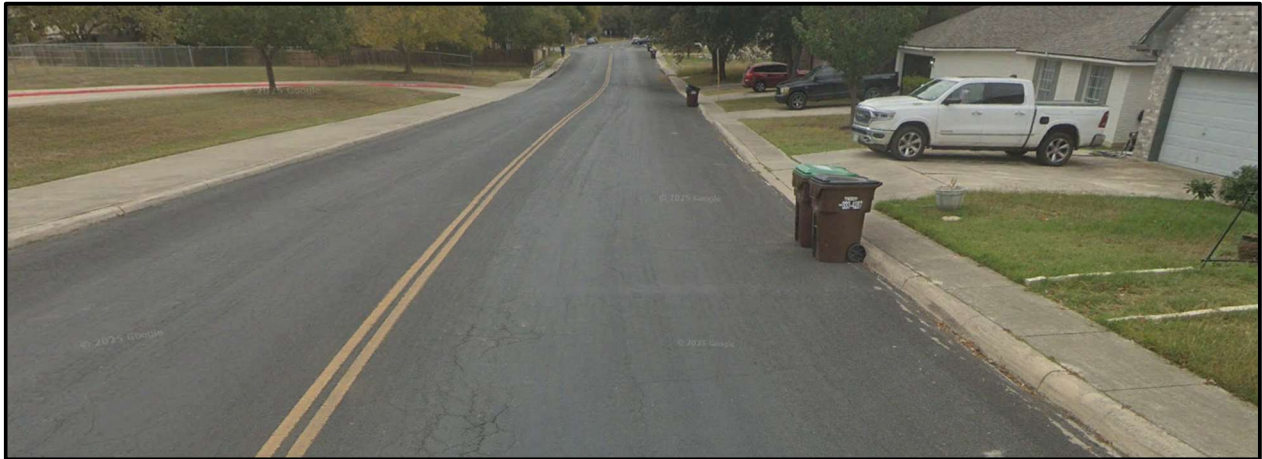
Figure 4 – Misty Ridge Drive Facing East
